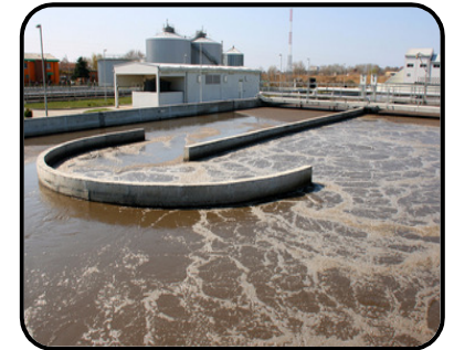
Water Treatment Plants
