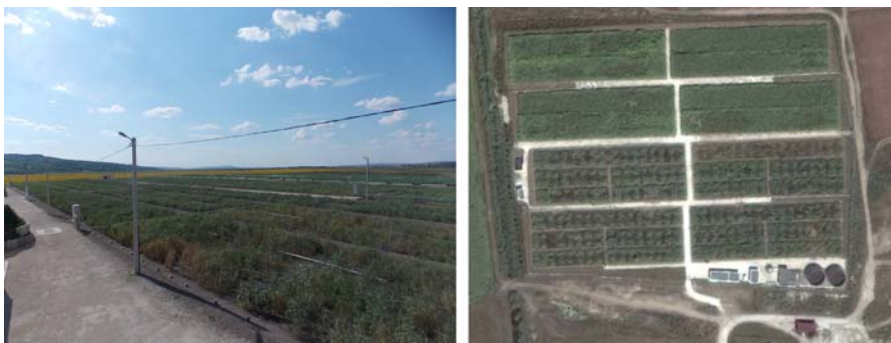
Figure 6.9 Case study 7 – Orhei Wastewater Treatment Plant (Moldova).
