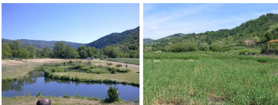
Figure 6.8 Case study 6 – Dicomano Wastewater Treatment Plant (Italy).
