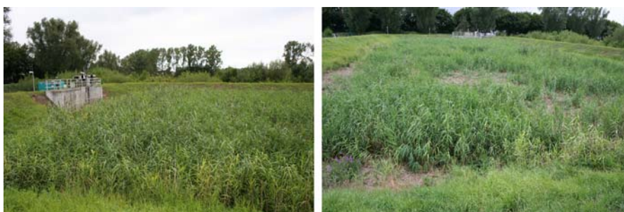
Figure 6.1 Case study 1 – CSO treatment wetland (Germany).
