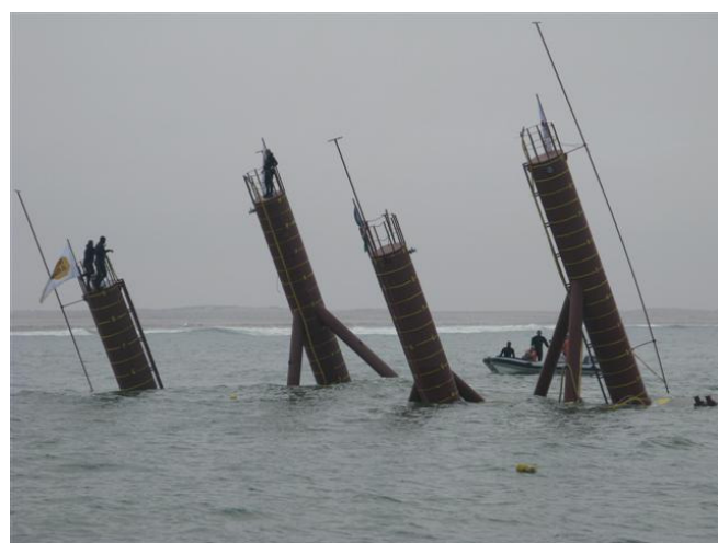
23 November 2008 (Being sunk at intake location)
