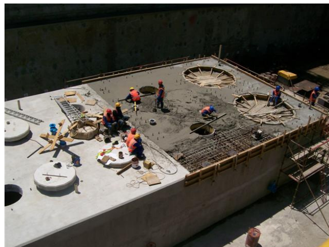
4 November 2008: Final concrete cast
