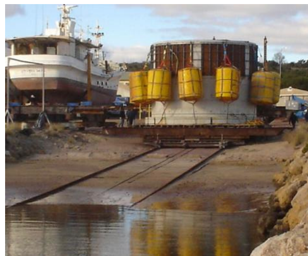
Installation of intake structure (Tom Pranktz)
