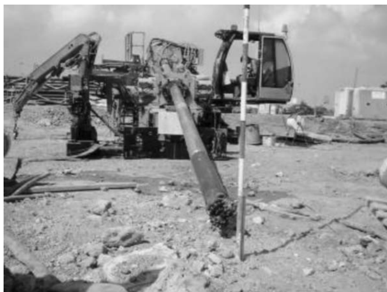
Fig. 16. View of the drilling rod and machinery.
