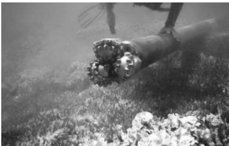
Fig. 18. The drilling head emerging in the sea from the sea bed.
