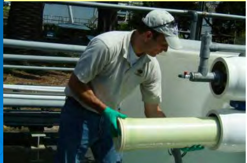
Standard 8" RO Membrane Element
