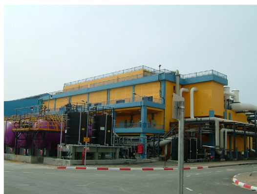
Fig. 4. Calcite contact tanks for the Ashkelon SWRO Plant in Israel (left hand side); Schematic of the \text{CO}_2 based calcite dissolution process (right hand side), as applied in the Hadera desalination plant in Israel. Final pH adjustment can be achieved either by \text{CO}_2 stripping or by NaOH dosage.
