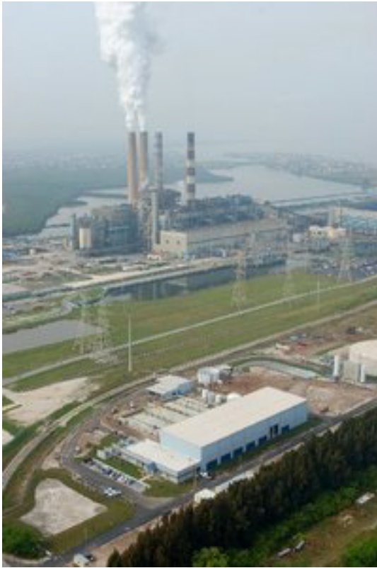
Figure 4-8. Aerial View of a Desalination Plant (foreground) Co-Located with a Steam Electric Power Plant (background) (TBW, 2008)
