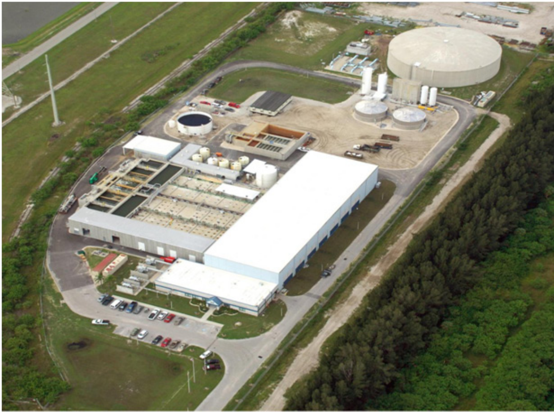
Figure 3-4. Tampa Bay Water Desalinization Plant (TBW, 2008)
