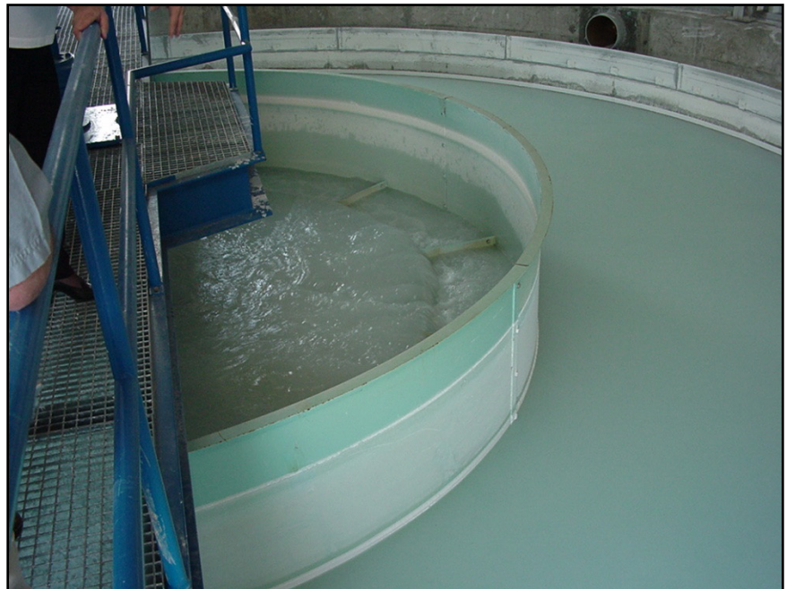
Figure 3-6. Post Treatment Lime Softening Using Slaked Lime
