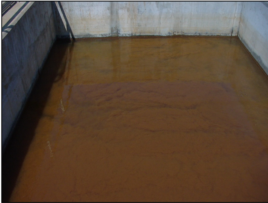
Figure D-2. Flocculation with Ferric (Iron) Chloride at the Tampa Desalination Facility (TBW, 2008)
