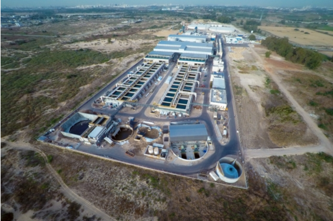
Figure 5.3: The Sorek desalination plant
