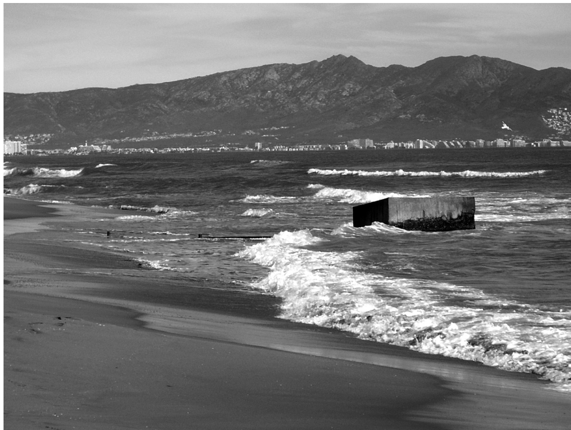
Fig. 2. Exposed part of an indirect seawater intake system (Photo: K. Peters, 2006).
