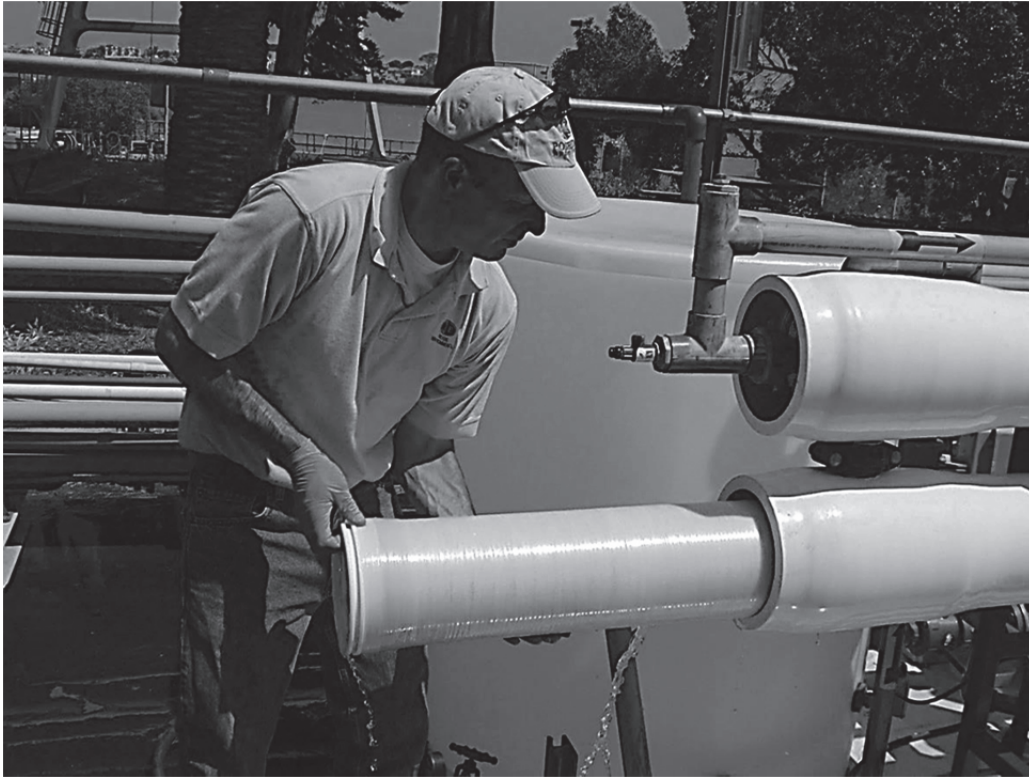
Figure 2.1. SWRO membrane element.
