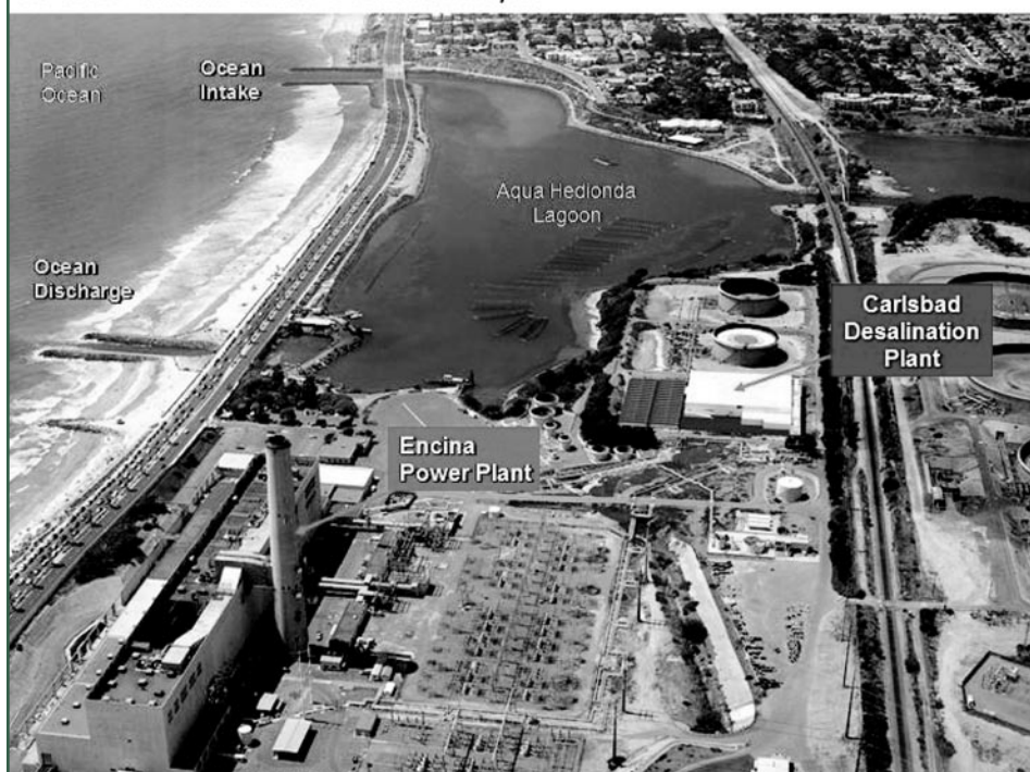
FIGURE 1 Carlsbad Sewater Desalination Project
