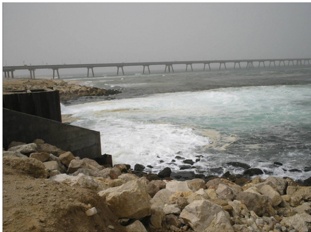
Fig. 6. Tidal zone discharge of the Ashkelon SWRO Plant, Israel.
