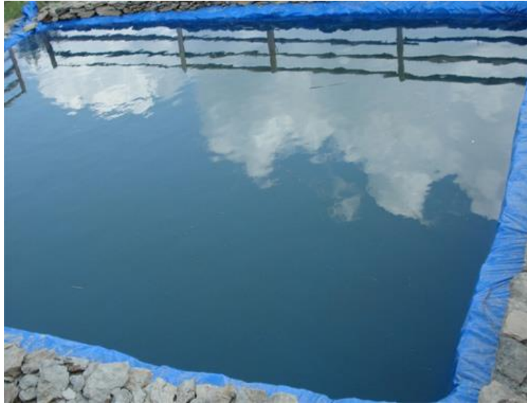
Water storage tank in each cluster
