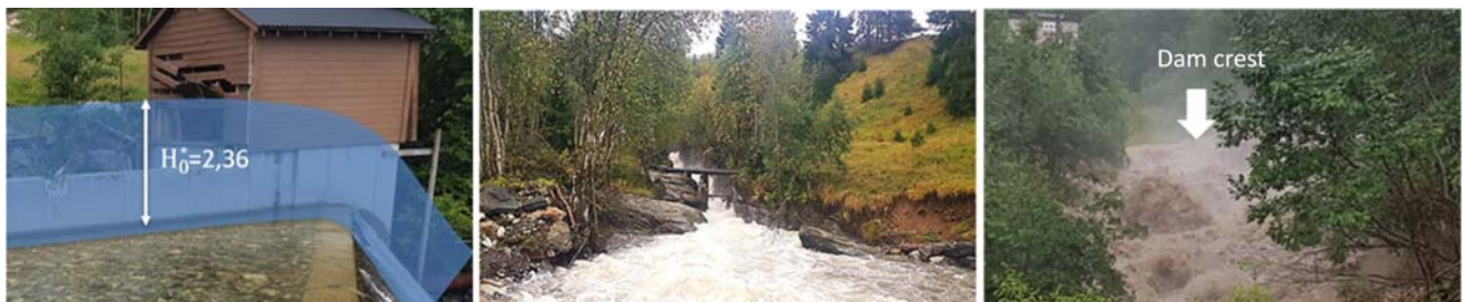
Figure 6 | Illustrated water over the crest level, and picture of upstream of the crest and of the flow over the crest during the event.
