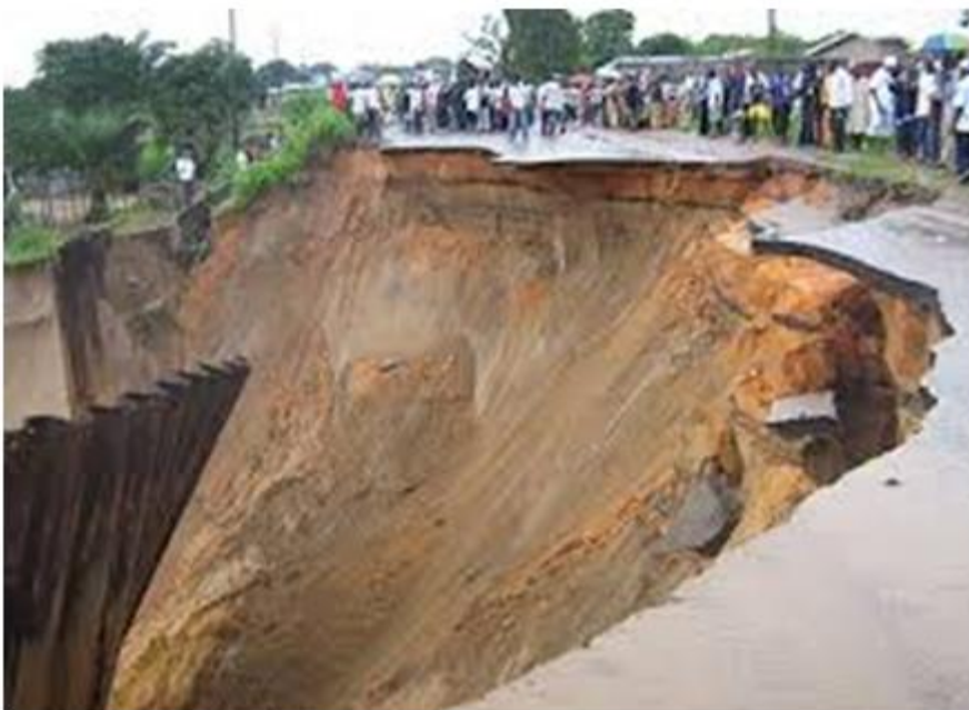
Erosion in Brazaville (Koua Stephen Faller, 2015)
