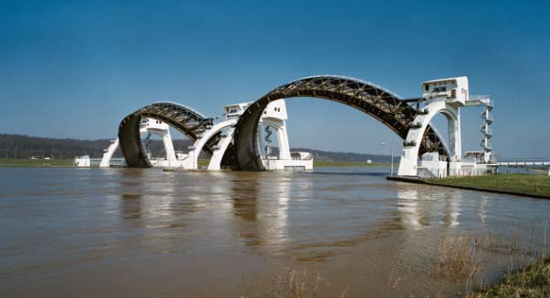
Weir in the Neder-Rijn at Driel.
