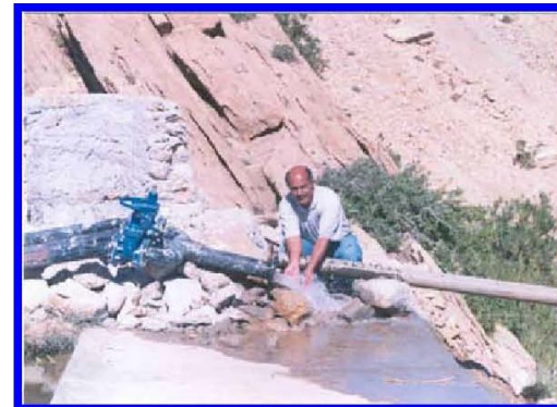
Water is flowing from a tap after priming the draining floater system
