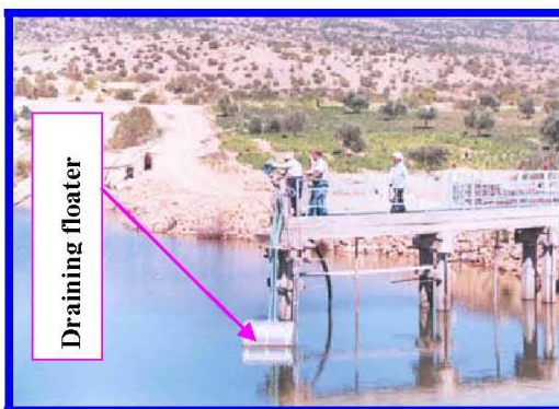
Attachment of the draining floater to a fixing system fixed to a footbridge
