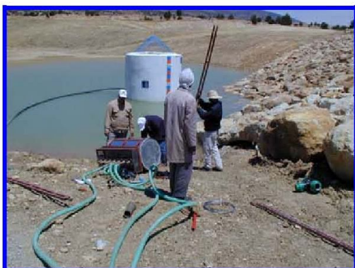
Connection of tubes to the floater and the tubes collector
