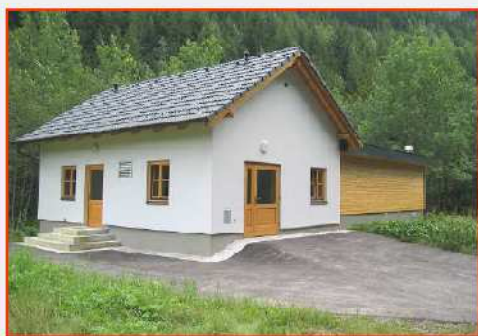
Waste Water Treatment Plants
