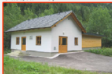
Classical PVS WWTP
