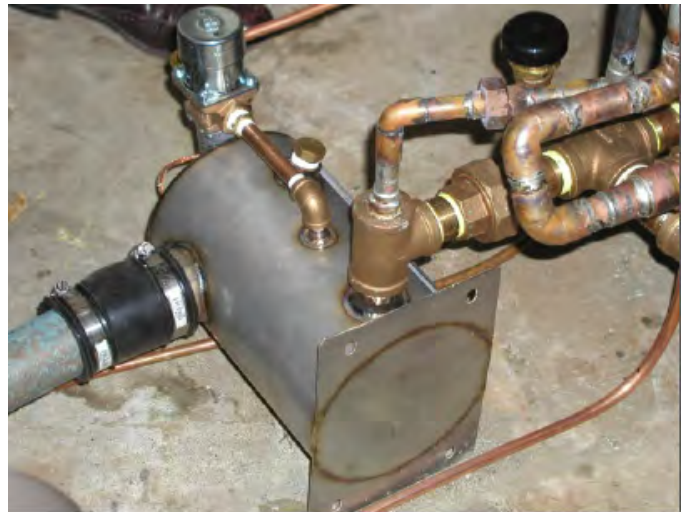
Example of a 'custom made' quench pot that is functioning correctly
