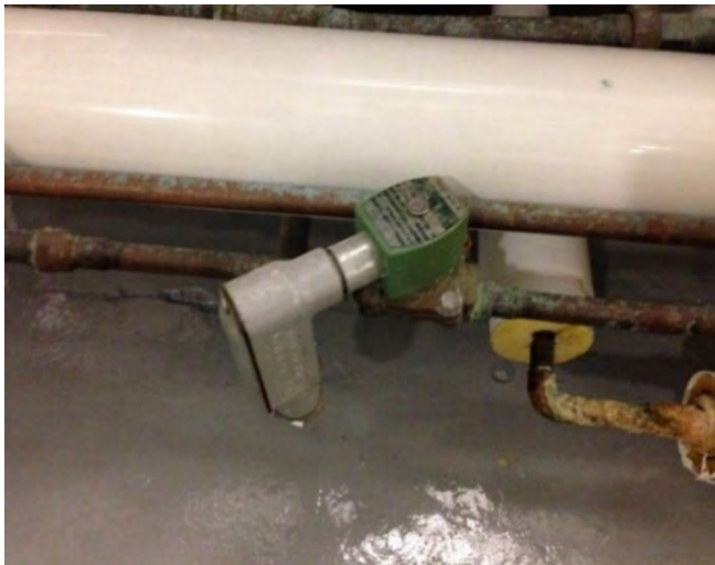
Solenoid on Amgen's city water 'quench' line that is failed
