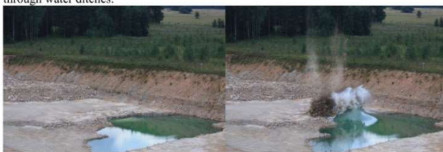
Figure 4 Underwater blasting
