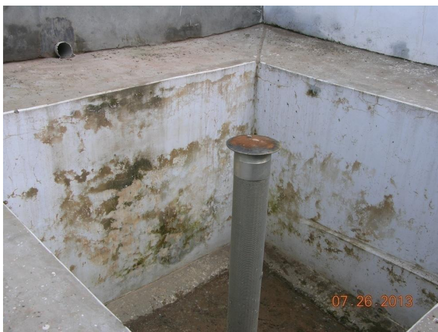
Fig. 9 Artificial Recharge Structure Constructed In Baddi University
