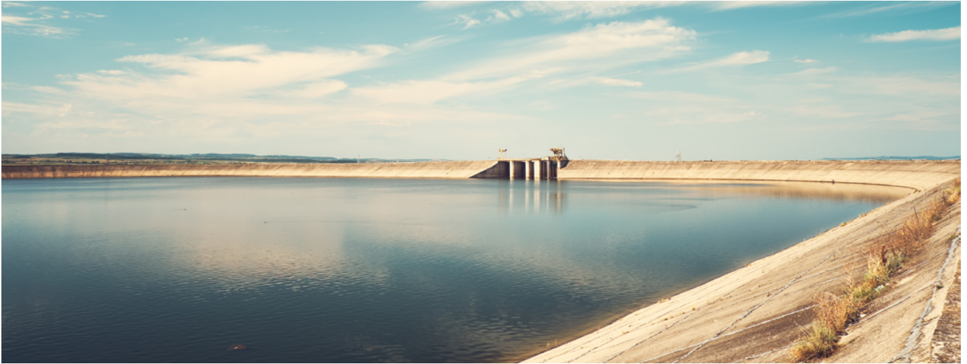
Figure 3: Drinking water reservoir.
