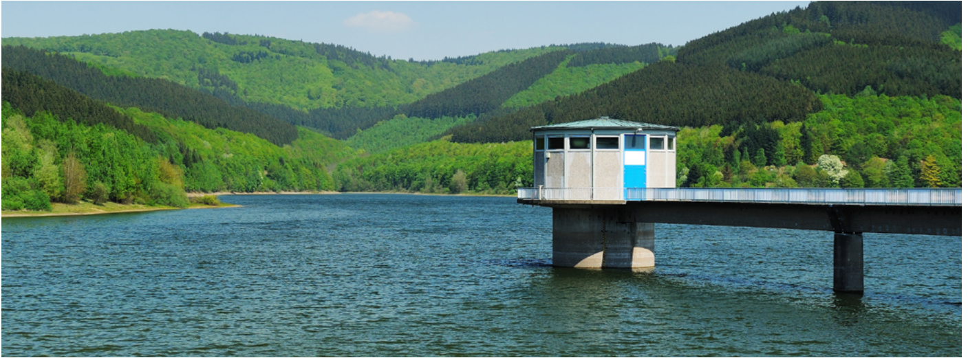
Figure 1: Drinking water reservoir.
