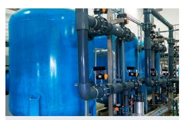
1,4-dioxane breaks through GAC filters more rapidly compared to other contaminants, resulting in reduced filter life and more frequent replacements of media.
