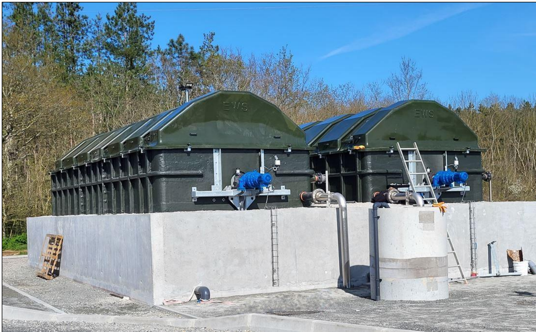
WWTP under construction – Capacité 800 PE – Two EWwS units
