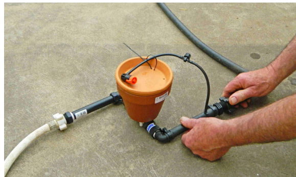
Connect the irrigation application to the outlet pipe
