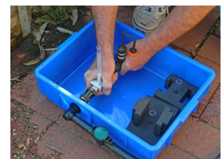
Float shaft must be vertical
