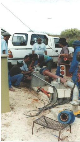
CMC staff assisting with installation for testing before treatment, Atlantis, 2002.
