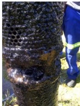
Photo 3: Pump from G30965, Witzands, 2014
