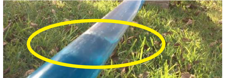
Figure 40. Baseline Disturbance from Re-Energizing Water Services.
