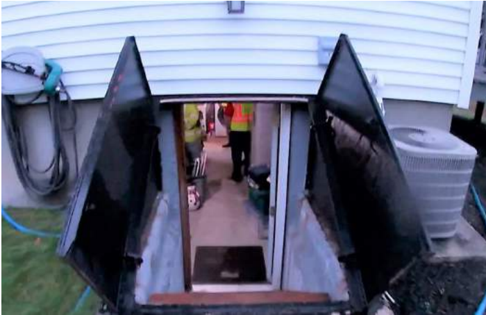
Figure 28. A Basement Entry in Massachusetts.
