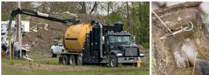
Figure 41. Typical Hydro Excavation Truck Used to Eliminate Topsoil.
