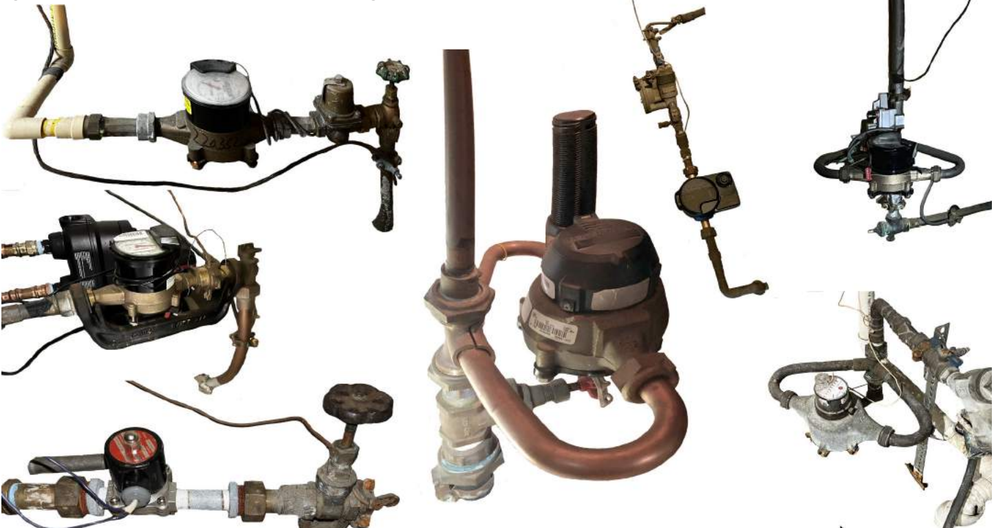
Figure 29. Various Basement Meters and Service Configurations.
