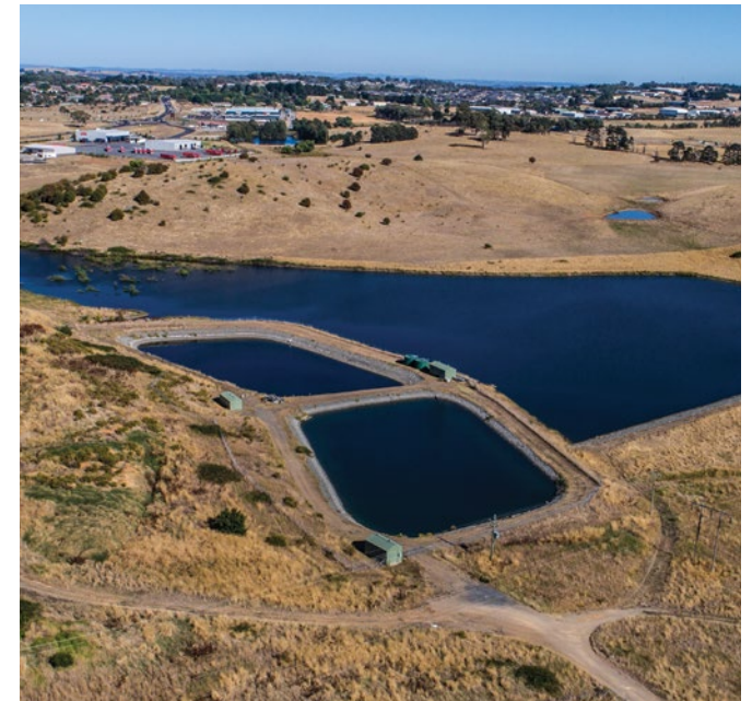
↑ Holding dam and batch ponds
