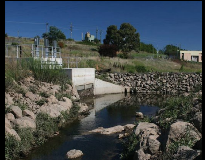
Blackmans Swamp Creek weir and harvesting pump station
