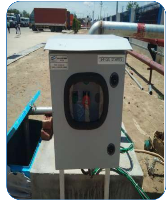
PUMP, STARTER PANEL CONNECTION
