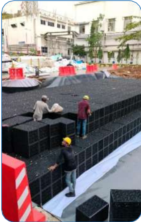
UNDERGROUND STORE & REUSE TANK
