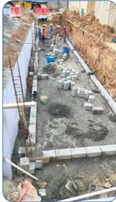
UNDERGROUND STORE & REUSE TANK
