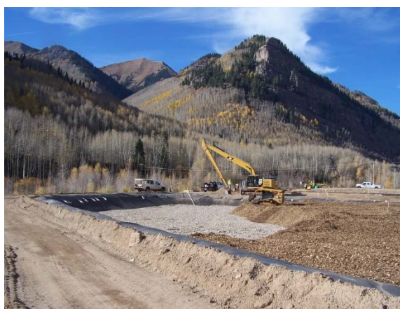
Figure 6. Installing biocell substrate, Rico Argentine EWD system, 2015.
