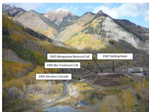
Figure 4. Annotated aerial photo of Rico Argentine EWD system, 2015.
