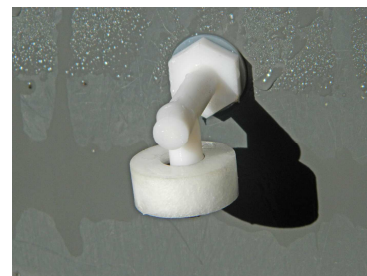
Float switch on the inside of the header tank with the float shaft pointing down
