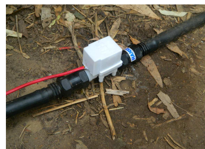
Solenoid valve installed at ground level
