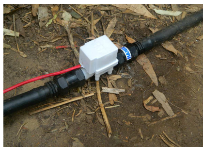
Solenoid valve installed at ground level
