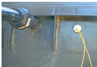
Float switch on the header tank is lower than the inlet
