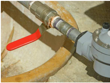
Connect the inlet of the solenoid valve to the water supply
