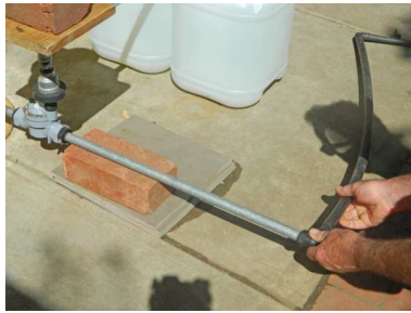
Connect the outlet of the solenoid valve to the irrigation application
