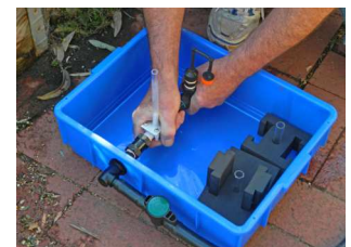
Float shaft must be vertical
