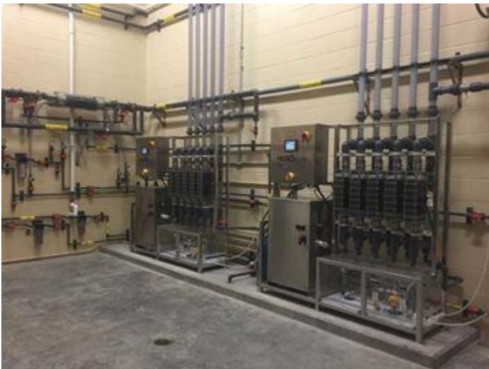
600 ppd Microclor® On-Site Hypochlorite System
