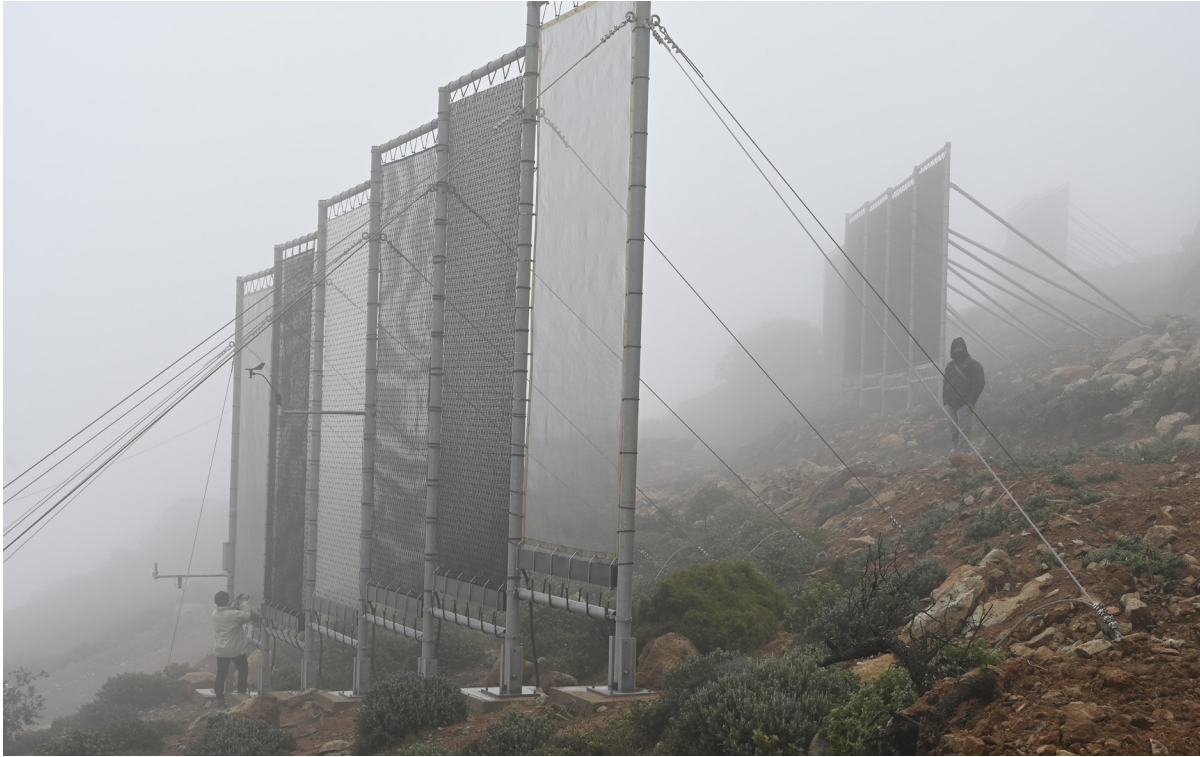
Figure 1 Fog water collection systems (Credit: Aqualonis).
