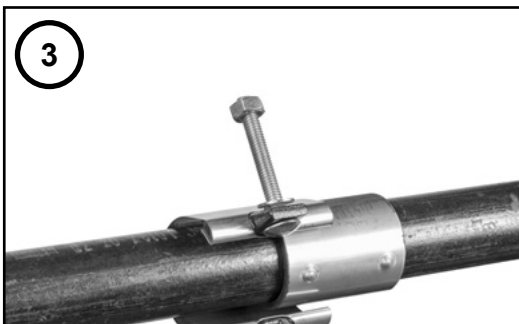
Step 3. Wrap the clamp over the gasket assembly.
