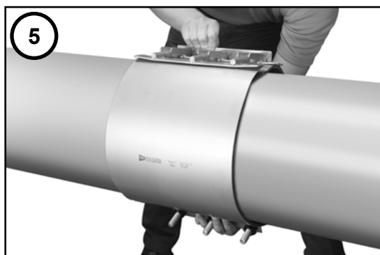
Step 5. Install on damaged pipe
