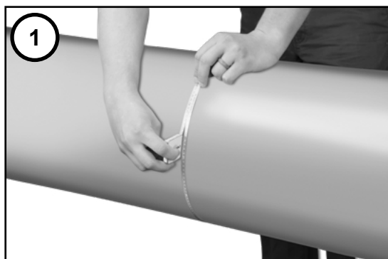
Step 1. Measure actual O.D. of damaged pipe with the provided O.D. tape measure.
