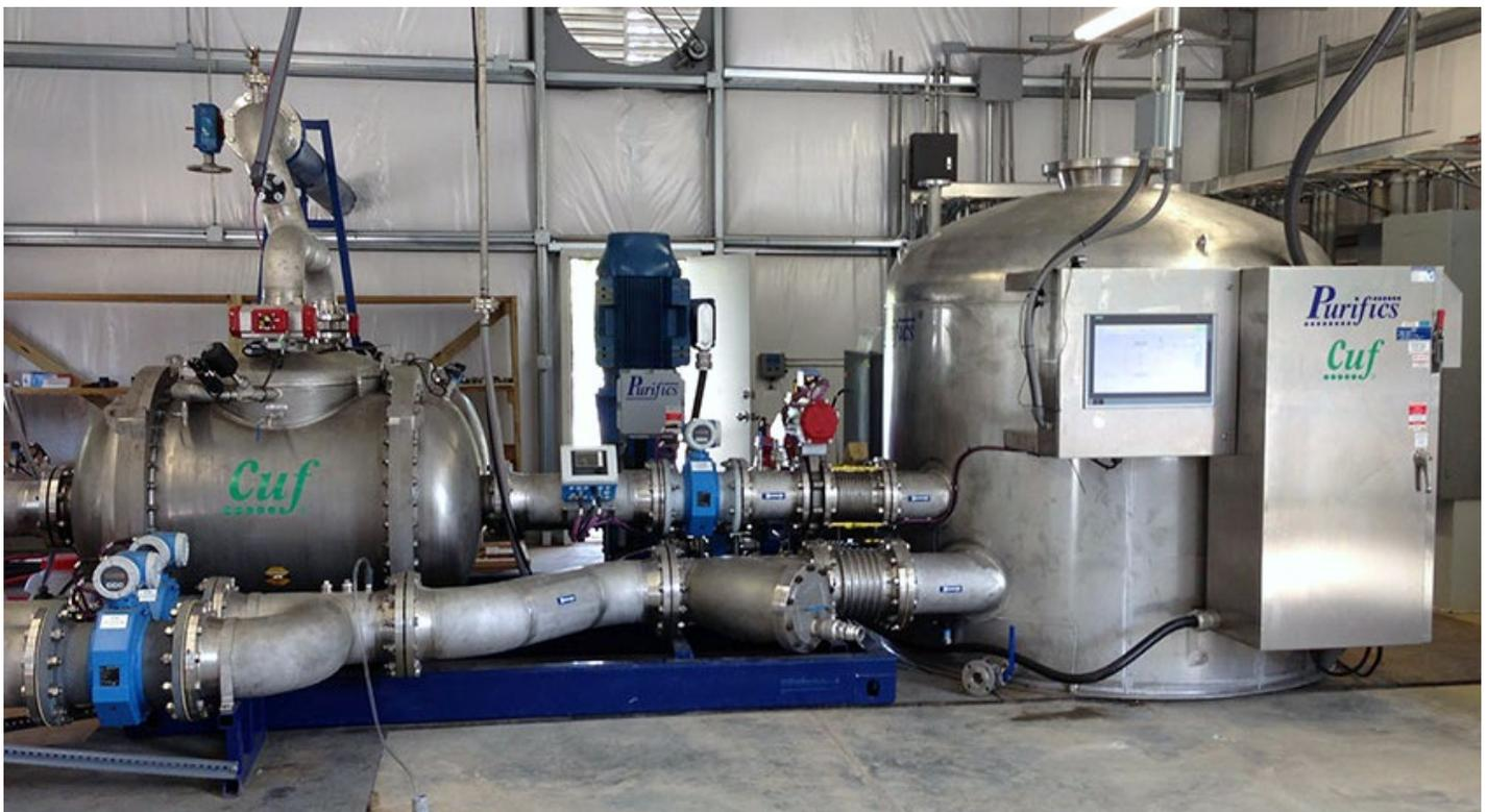
The palletized *Cuf* above is the entire water plant and operates on demand removing Color, Fe and the majority of DOC which significantly reduces chlorine demand. Accordingly, once the *Cuf* system was brought on-line chlorine addition was reduced by 75%. Reduction in DOC and chlorine residual solves THM & HAA formation problems. Purified water is discharged directly to the clear well.
