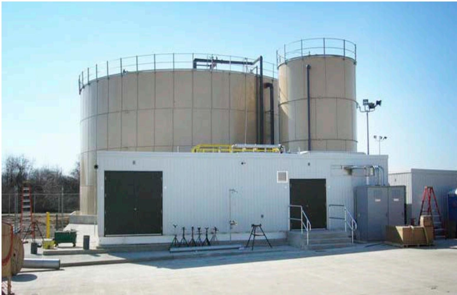
Membrane Bioreactor System
