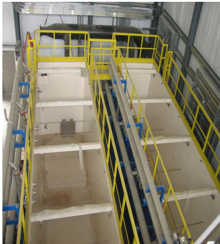
Steel (Above Ground) Membrane tanks
