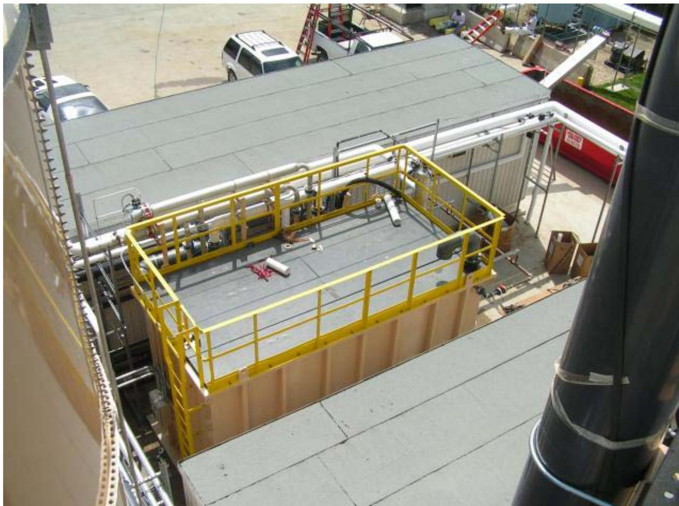
Steel (Above Ground) Membrane Tank
