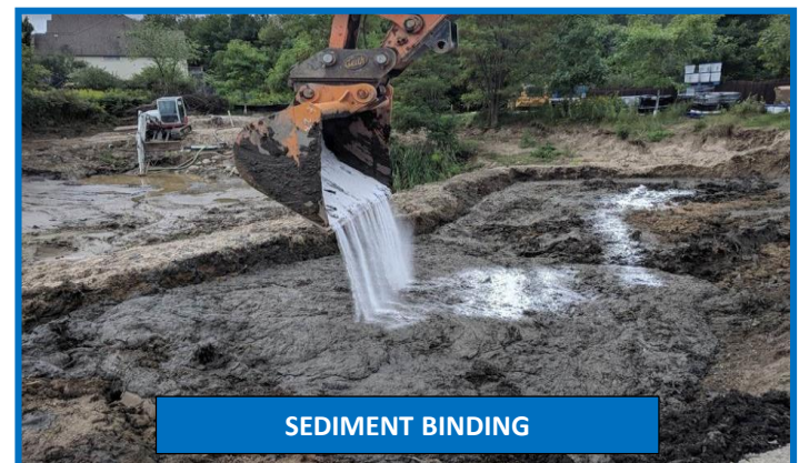
DEWATERING AND TSS CAPTURE
