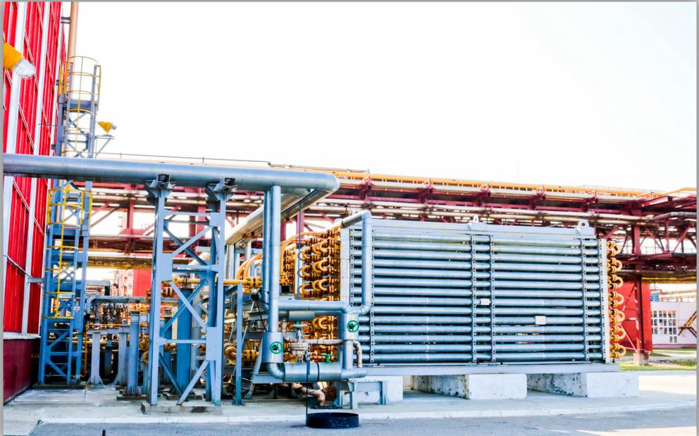
PHT-Ox reactor treats the high COD wastewater using proprietary catalyst and Oxygen. It consists of Plug Flow Reactor on a prefabricated skid.
