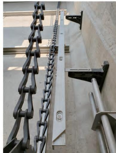
Collector chains, Head sprockets, Driven sprockets, Take up sprockets
