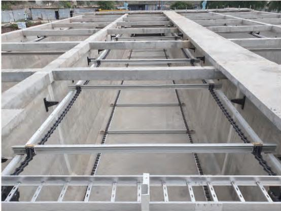
Flight will be made of G.R.P. which is drawn construction to avoid crack and maintain high strength. GRP has been reinforced by high strength of fiber glass by 50% and absorbing rate is less than 0.5%. Mostly installed by 3m of interval
