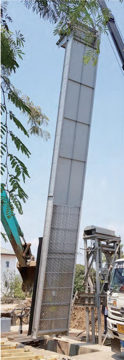
Installation of fine mechanical bar screen
