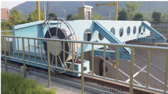
Submersible sludge scraper driven by stainless steel wires
