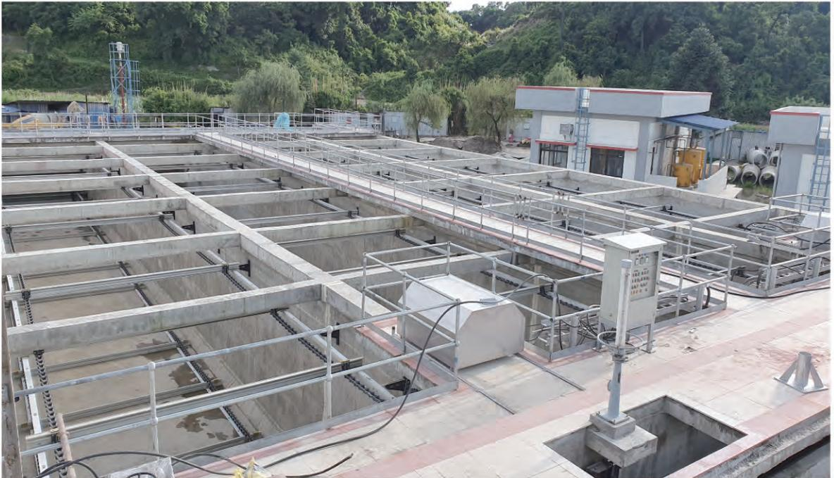
Non-metal sludge collectors, 8 units for primary sludge settling tanks, and 4 units for secondary sludge settling tanks, supplied and has started run by DWA in Kathmandu, Nepal in 2018 to 2019. Dimensions are 23Lx5Wx3.5Hm and 40Lx4Wx3.5Hm
