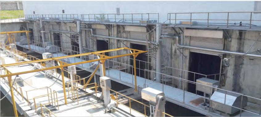
6 Band screens are installed in potable water treatment plant in Korea
