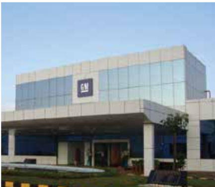
General Motors, Talegaon Pune
