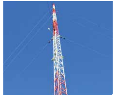
470m High Guy Mast Communication Tower
