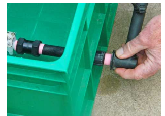
Attach the adjustable control dripper assembly to the outlet pipe
