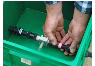
Connect the inlet pipe to the valve assembly
