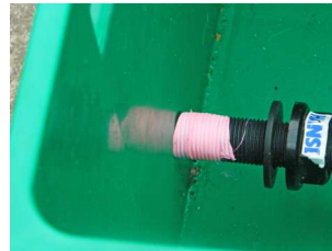
Wrap teflon tape around the inlet and outlet pipe
