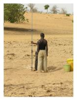
A screw is turned into the ground by successively adding more drill pipes to the top of the string. After a few turns, the entire drill string needs to be removed for emptying. Not suitable in gravel, rock, or collapsing ground. Sometimes used to reach the water table before changing to another manual method, but rarely used for the entire depth of drilling.
