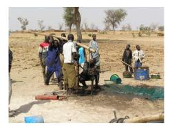
A steel pipe is raised and lowered in the borehole using a lever, while another crew member alternately covers and opens the top of the pipe with the palm of their hand. The hole is kept waterfilled. As drilling progresses, a slurry of water and drill cuttings is lifted in the drill pipe. A common technique in unconsolidated formations in Asia.
