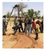
A set of heavy tools suspended by a rope (manual percussion) or a cable (machine drilling) is successively raised and dropped to break ground and, with some tools, grab spoil. The tools need to be lifted for emptying. Suitable in many types of geology, but slow in hard rock.
