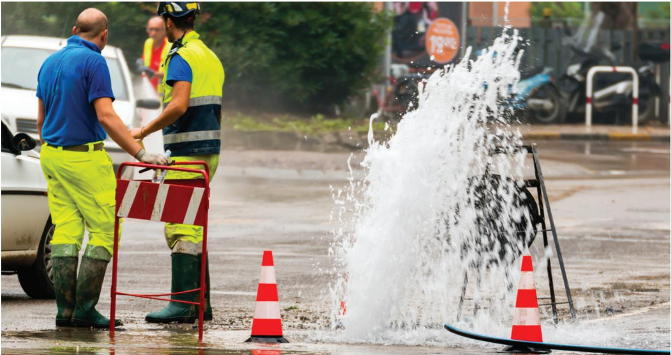
Using the equations in Figure 34 with  $x=1$  for a low corrosion risk and  $x=3$  for a high corrosion risk, one can show that a cast iron pipe in a high corrosion soil is expected to have over 20 times the break rate of one in a low corrosion soil. Similarly, ductile iron pipe in a high corrosion soil has over 10 times the break rate than one in a low corrosion soil. Very poor correlations were found for the other material types in this survey.
