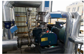
Lobe Compressor for evaporation upto 2T/hour
