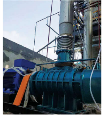
Lobe Compressor - For low capacity eveporation
