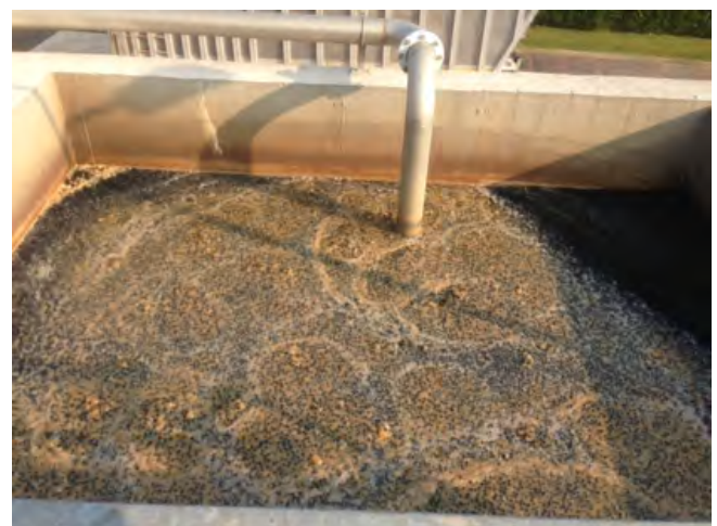
Figure 37: MBBR Media carriers in an Italian steel plant
