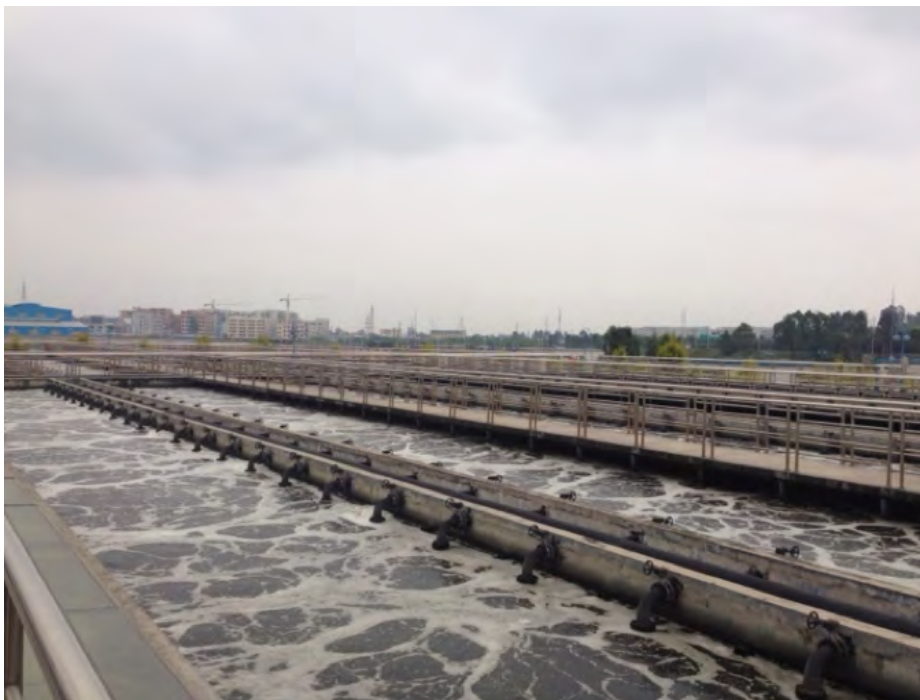
Figure 30: Aeration tank in a textile effluent treatment plant in China
