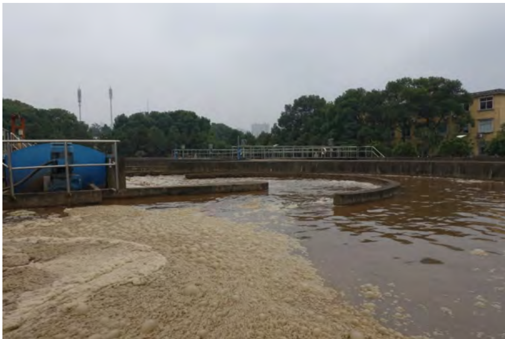
Figure 32: Photo of an oxidation ditch, China
