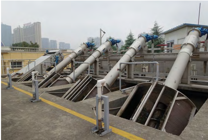
Figure 13: Fine screens in a sewage treatment plant
