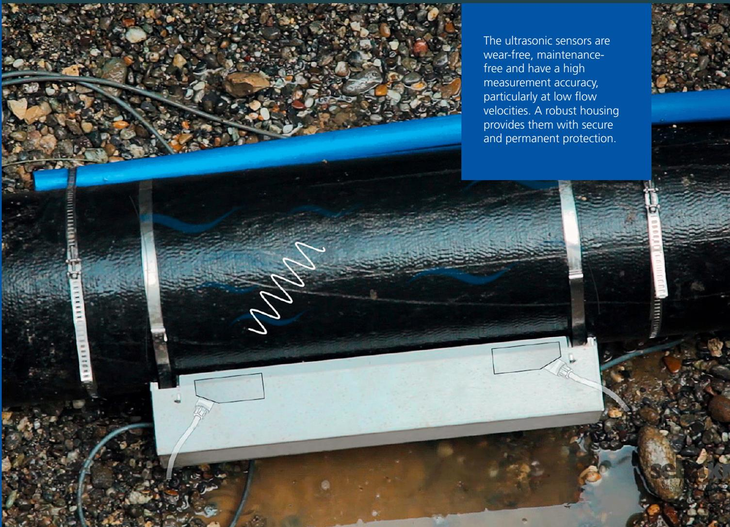
The ultrasonic sensors are wear-free, maintenance-free and have a high measurement accuracy, particularly at low flow velocities. A robust housing provides them with secure and permanent protection.
