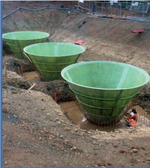
The base cones of 3 settlement tanks await assembly of the upper part. Arthurstown WWTP – Ireland
