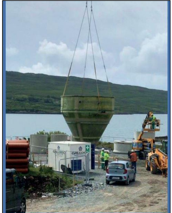
Handling of a 6m diameter settlement tank before installation
