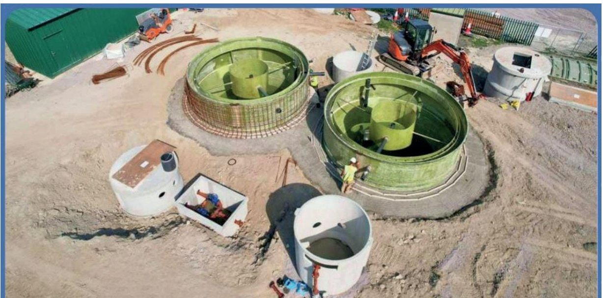
Two 6m diameter settlement tanks under construction
