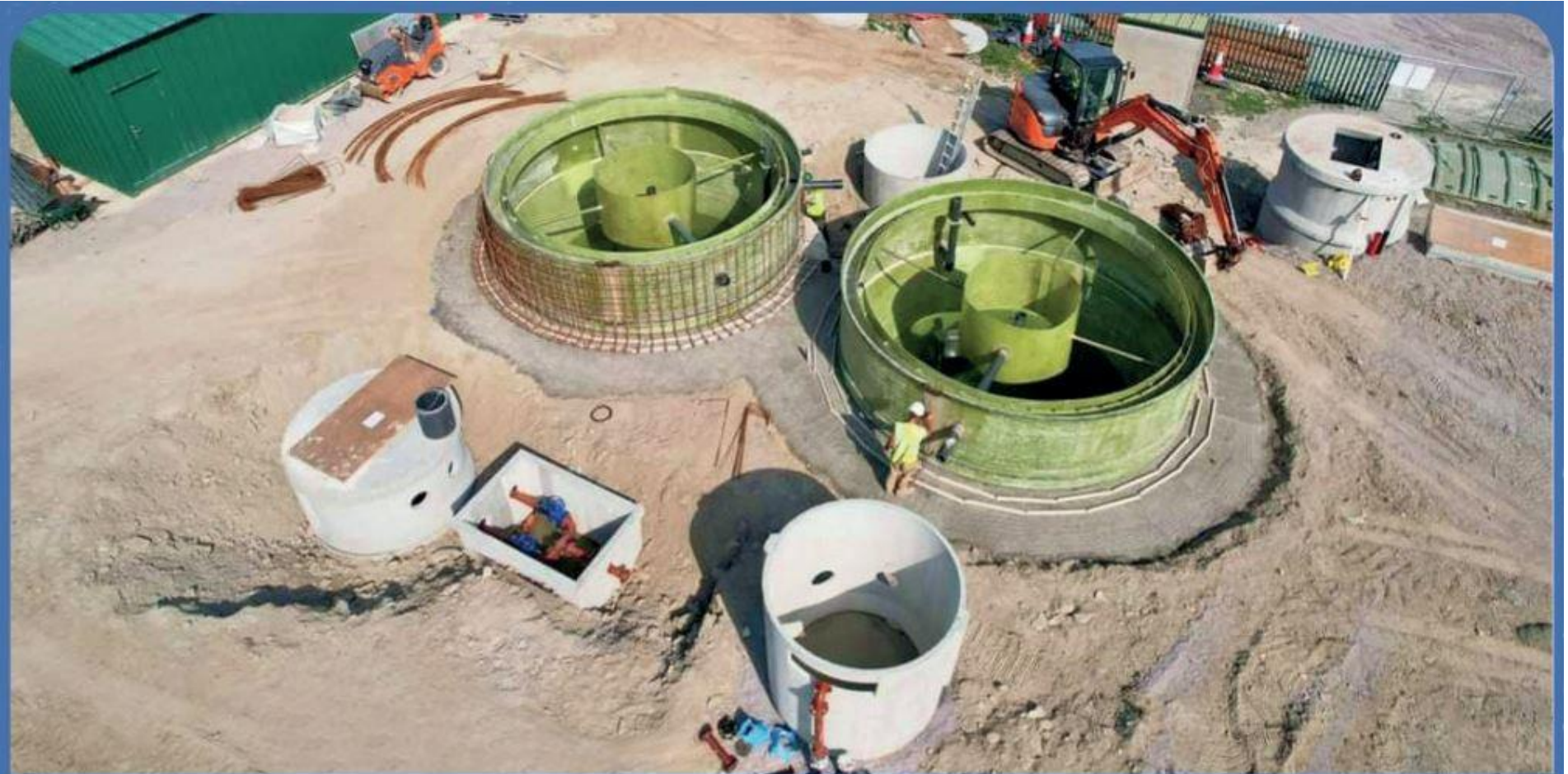
Two 6m diameter settlement tanks under construction
